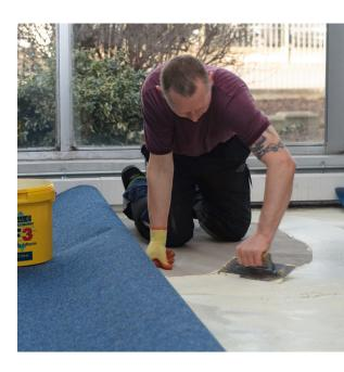
Essentially, the sub floor should be clean, dry and free from contamination such as dust, with any loose material cleaned by scraping, brushing or vacuuming the surface. Contaminants such as paint, residual adhesives, oil, mould or mildew should also be removed using appropriate cleaning products and methods, as they can all prevent adhesives from bonding properly.
